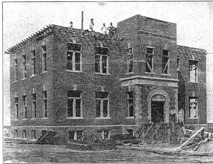
NEW HIGH SCHOOL—Under Construction
